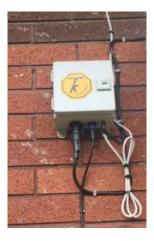
The Power Portal requires a 100V to 240V AC mains supply at 50/60Hz, 1.2 Amp, and provides 12 Volt power and internet connection to iVIBE, iDB, iGAS, iDUST and other instruments
